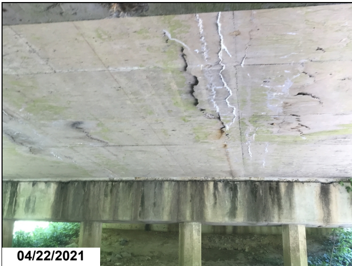
Span 2 near center line at mid span has large delam with staining.
