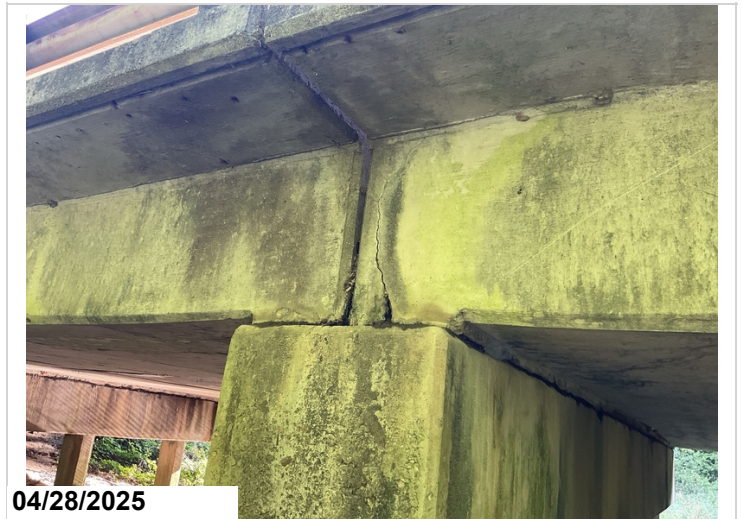
Span 1 Bent 2: Vertical crack/ delamination in side face of slab/deck.
