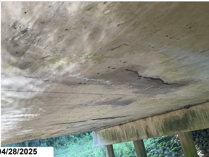
Undersurface Span 2: Large delaminations with staining.
