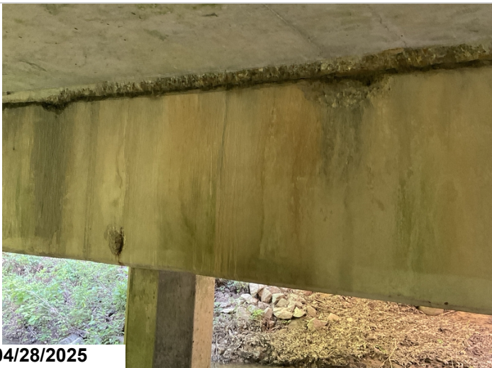
Cap Bent 2 Back: Small spalls and exposed rebar.
