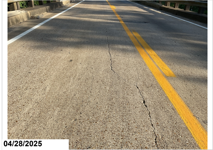
Deck Span 1: Large unsealed cracks.
