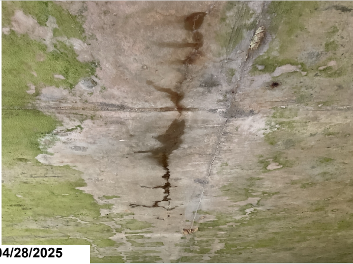
Undersurface Span 1: Large cracks with staining.
